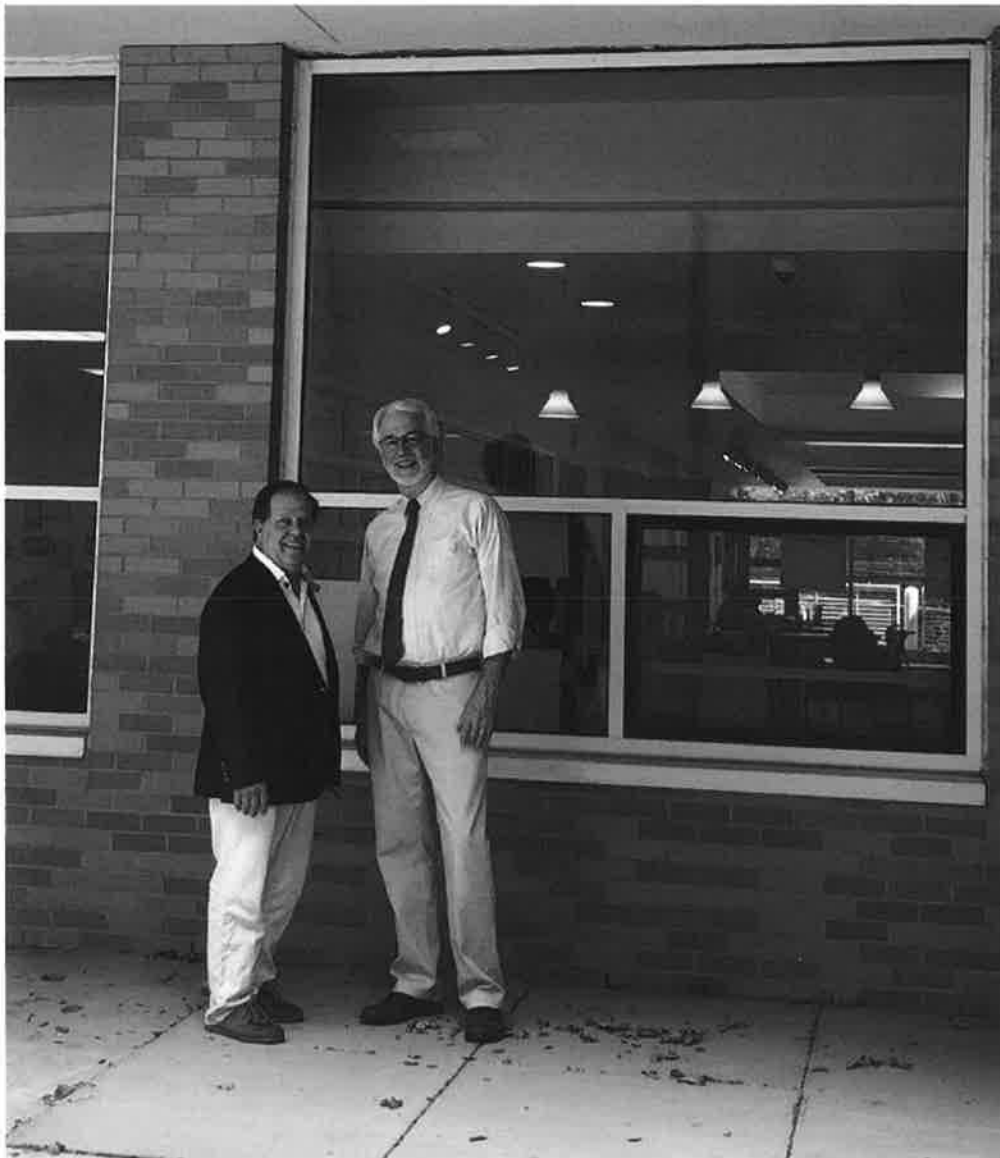
This outdoor space will soon become an enclosed “eating room” / café for Greenburgh Public Library thanks to a $143K grant from the State of New York and funding from private donors.
